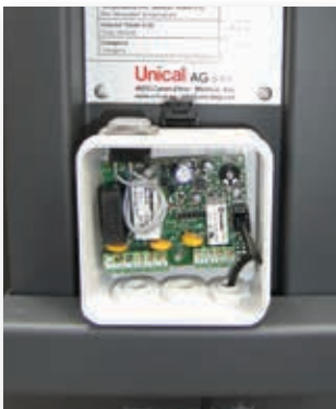
■ Temperature regulation system, with NTC sensor
