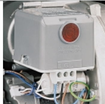
Control box fitted with an ignition transformer
